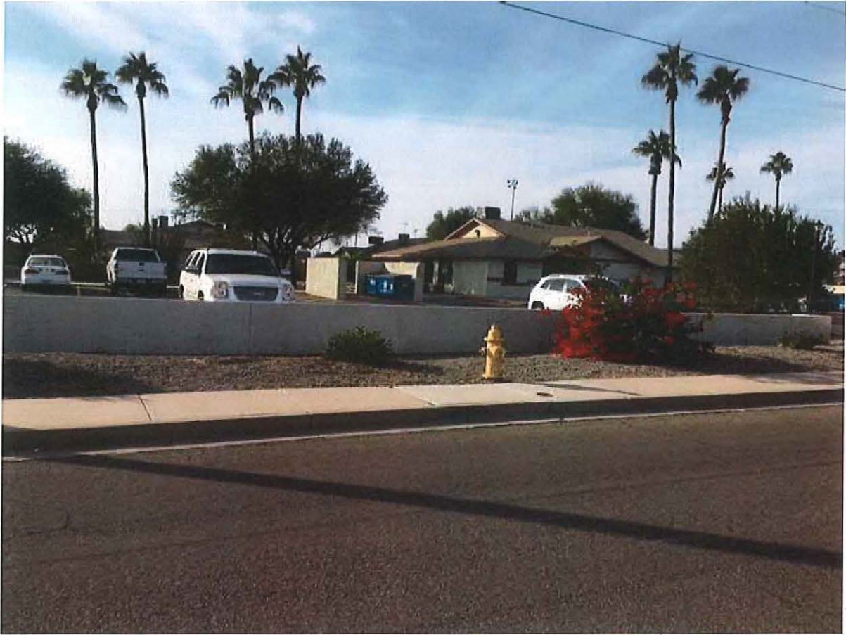
Figure 3. Buckeye Senior Apartments 605 S. 4th Street
